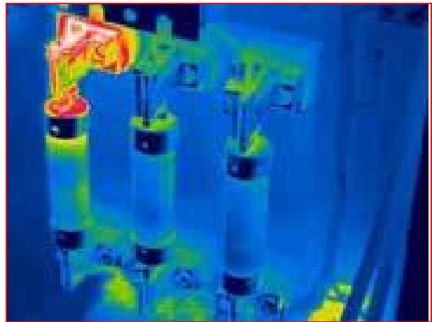
Fig. 11: Thermal image of a local hotspot in the hydraulic system
